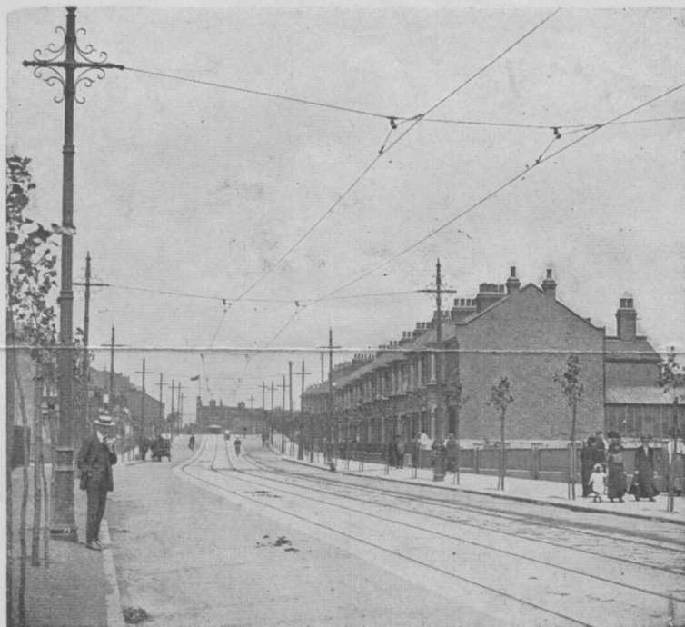
SPAN - WIRE CONSTRUCTION.
